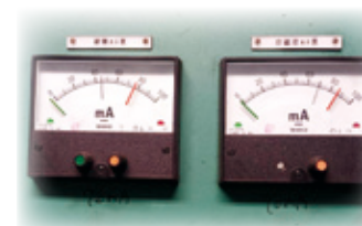
Monitoring Equipment for Coil Cooling Water Temperature and Leakage Current ▲
