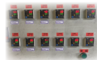
Monitoring Equipment for Coil Cooling Water Temperature and Leakage Current ▲
